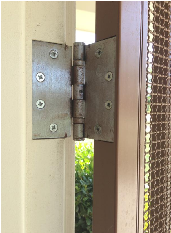
Properly Installed Gate-Frame Hinge
