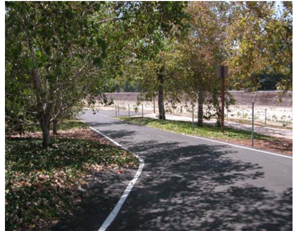
The San Diego Creek Trail is predominately asphalt and has shoulder striping along most segments.
