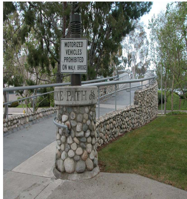
Approach to an overcrossing of Barranca Parkway, within Woodbridge. The overcrossing allows trail users to move from a residential area on the north side of Barranca Parkway to a shopping center and a connection to the San Diego Creek trail on the south side, without navigating through traffic or having to move east or west along Barranca Parkway to reach a controlled intersection.
