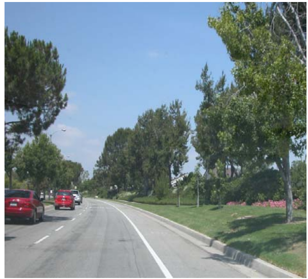
A typical Irvine Class II bicycle lane is located along an arterial with no curb-adjacent parking and built to a width compliant with Caltrans Highway Design Manual, Chapter 1000.
