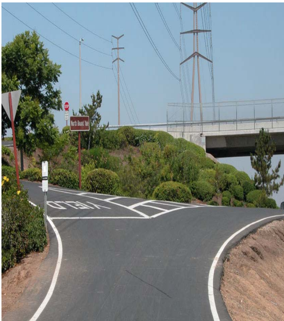
A typical approach to an arterial undercrossing; to the left a trail user can approach Yale Avenue at grade, while to the right a trail user can cross underneath Yale Avenue unimpeded by automobile traffic.
