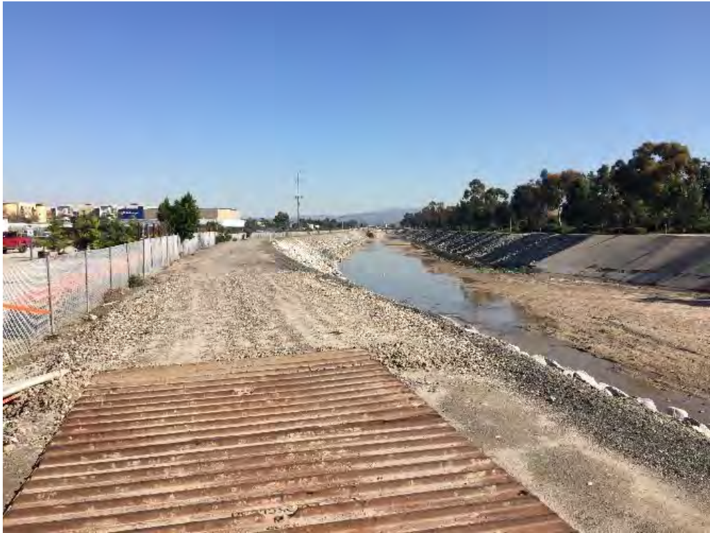
Segment 4 north of Main Street facing north
