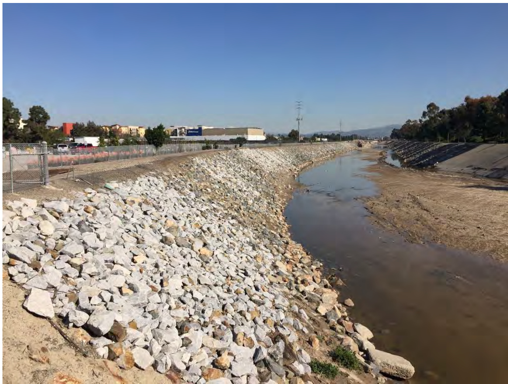
Segment 4 on Main Street facing north
