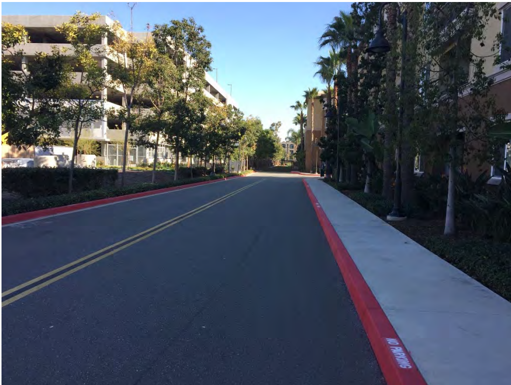
Segment 7 north of Main Street facing north
