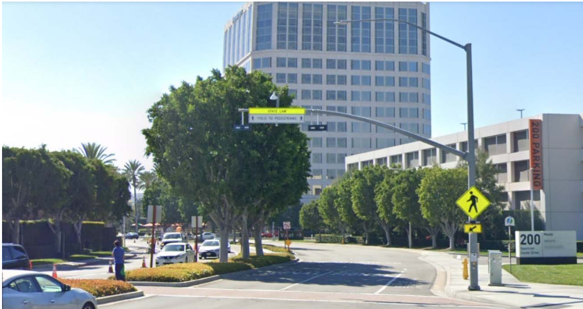
Spectrum Center Drive at Quasar Drive facing south
