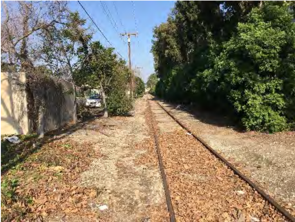
Segment 2 north of Alton Parkway facing north
