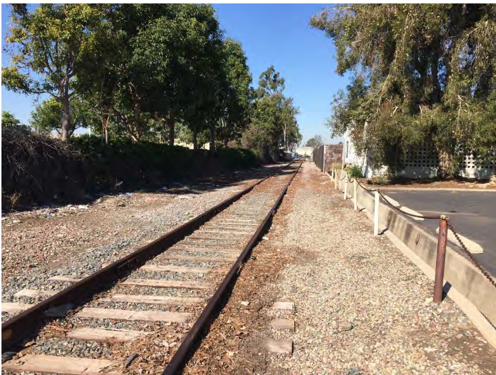
Segment 2 west of Red Hill Avenue facing west
