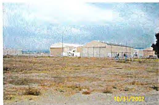
Former Location of ASTs and Pump House (Facing Northeast)
