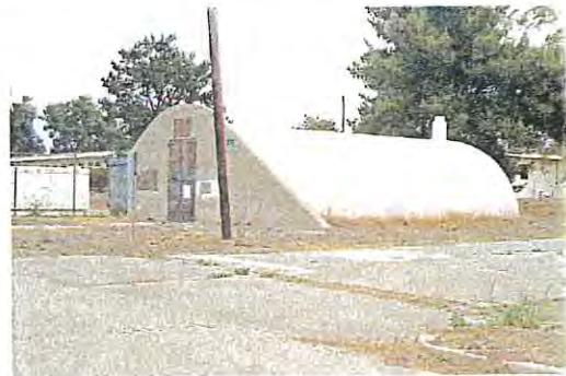
Exterior View of Building 165 (Facing Southeast)
