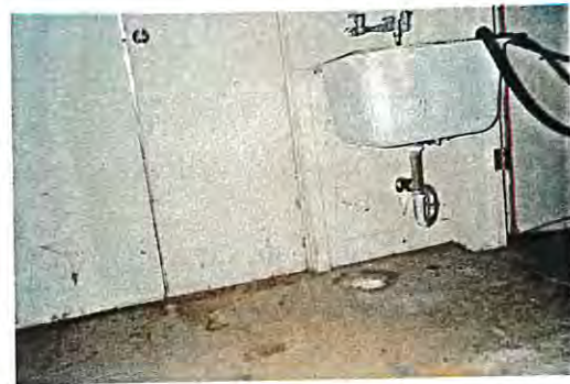
Service Sink: Drain Sample DS2 Collected From P-trap (Facing Northeast)
