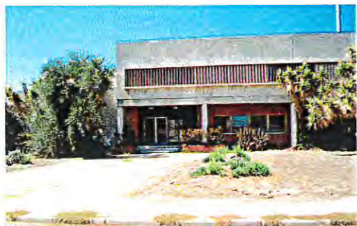
Exterior View of Building 443 (Facing Northwest)
