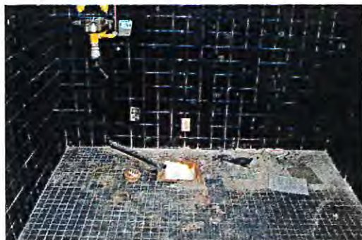
Dark Room with Floor Drain: Location of Soil Sample Boreholes HA4 and HA5. (Facing Northeast)
