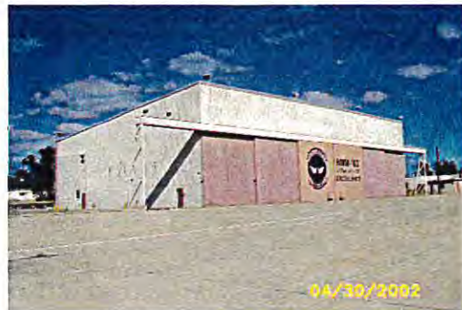
Front of Building (Facing East)
