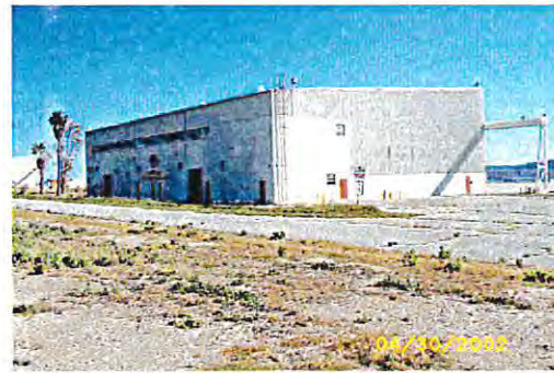
Northeast Corner of Hanger (Facing South)
