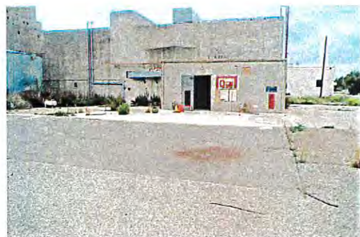
Exterior View of NW Corner of Building (Facing South)
