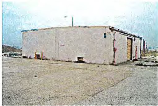
Building Exterior (Facing Northeast)
