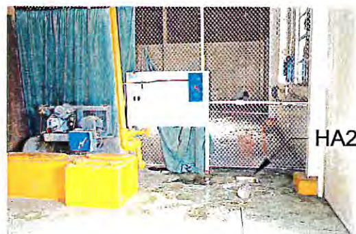
Photo of Area Near Borehole HA2. Air Compressor at Left and Floor Drain and Borehole at Lower Right of Photograph (Facing East)
