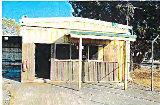
Front of Building 626 (Facing Southeast)
