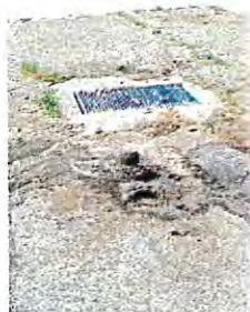
Soil Sample Borehole HA1 Adjacent to Storm Drain (Facing West)
