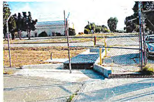
Trench Drain & Drainage Ditch at Entrance to Facility with Integrated Oil / Water Separator (Facing Southwest)
