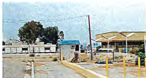
Former Fuel Dispensing Area with Remains of Remediation Piping (Facing Southwest)
