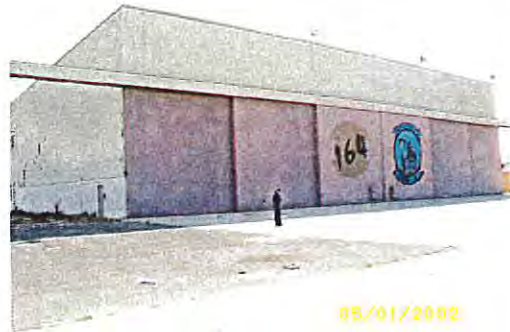
Building Exterior (Facing Southeast)
