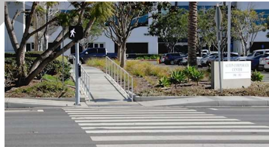
Pedestrian Hybrid Beacon Crosswalk, City of Irvine
