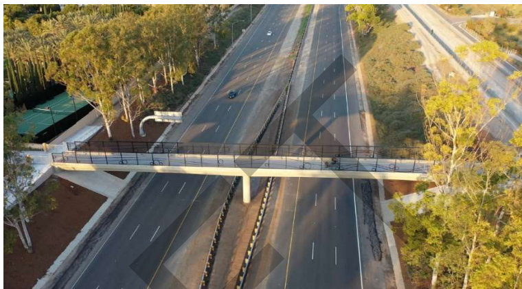
Venta Spur Bicycle-Pedestrian Bridge Aerial View
