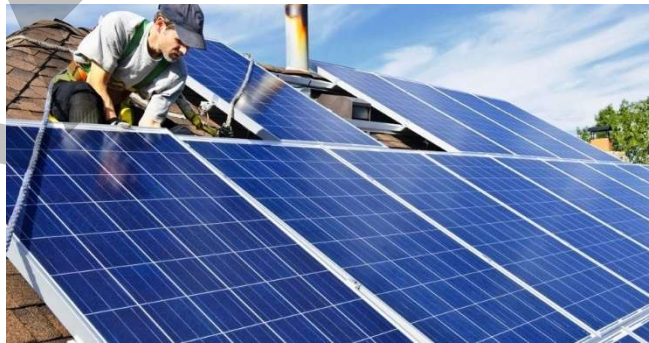
Rooftop Solar Energy System installation.
