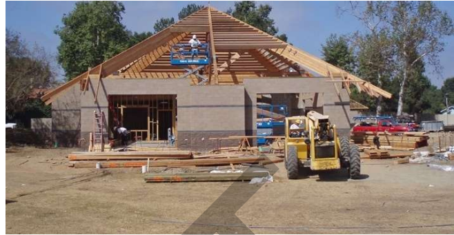
City of Irvine Construction Project
