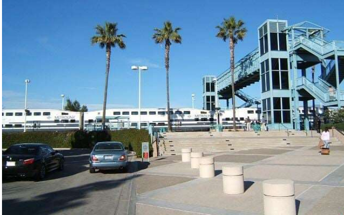
Irvine Train Station. Source: Metrolink
