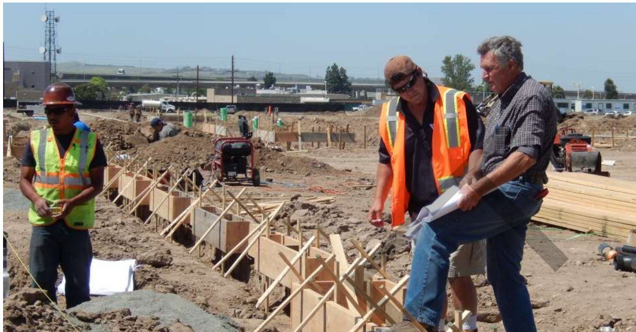
City of Irvine Building and Safety Inspection Services
