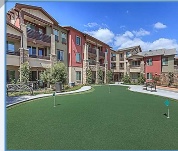
High Density (0 - 40 units/acre). Multifamily housing with on-site recreation areas for common use.
