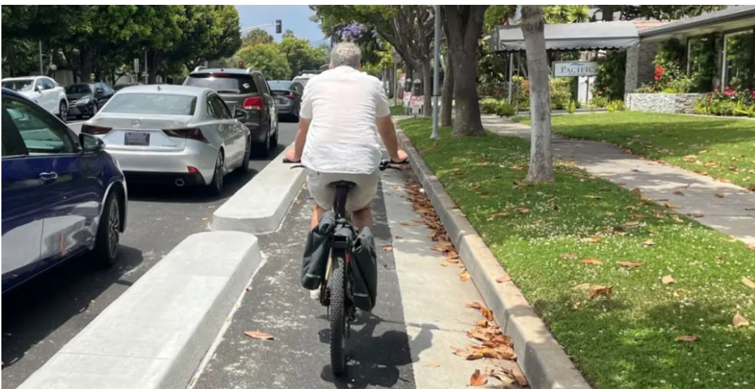
The City of Santa Monica used an extruded curb method to create concrete barriers along the bike facility on 17th Street.
