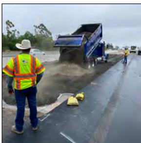
The project includes asphalt pavement restoration, adjustment of valve covers, pull boxes, and manhole covers to match the grade, replacement of damaged concrete curb, gutter, curb ramps, and installation of new signage and striping.
