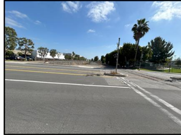
PHOTO 2: View looking northeast of the Barranca Channel parallel with a railroad along McGaw Avenue.
