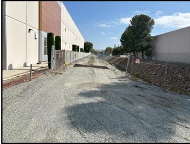
PHOTO 1: View looking northeast of the Barranca Channel surrounded by industrial uses along Alton Parkway.
