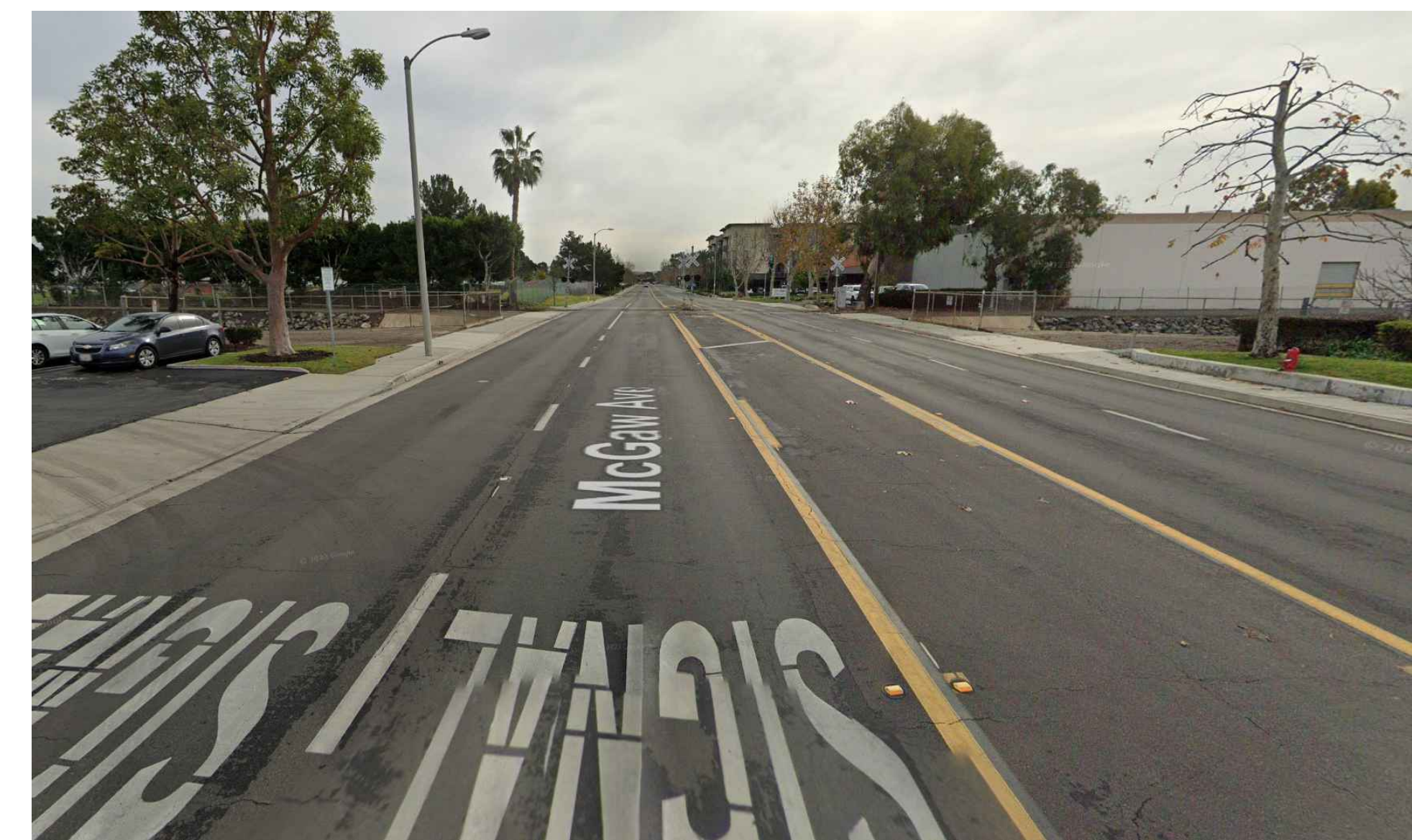
VIEW ON MC GAW AVENUE, FACING EAST
