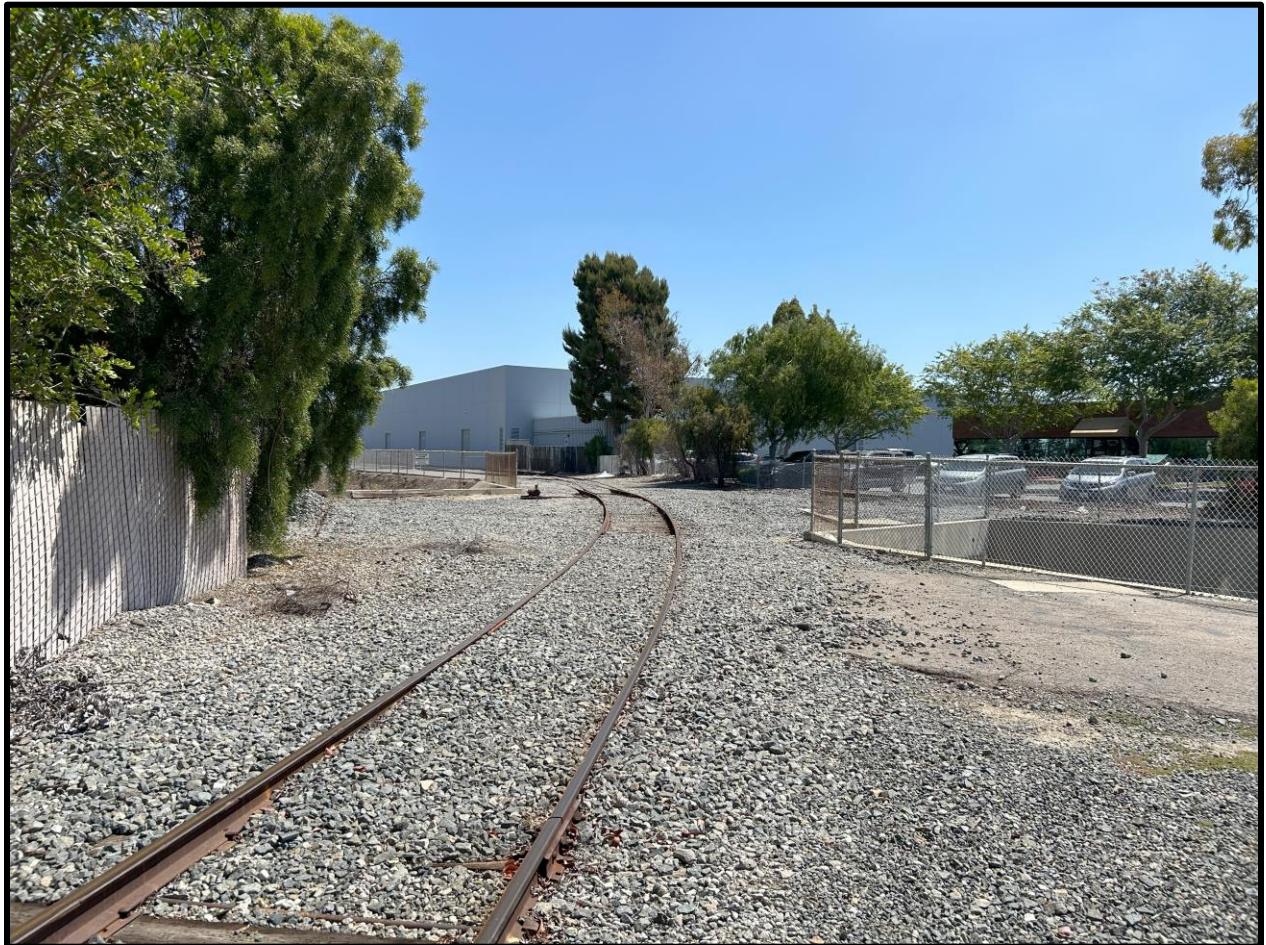
Figure 4.3-6 RAILROAD TRACKS AND BRIDGE CROSSING FROM WEST BANK OF BARRANCA CHANNEL IN THE MCGAW AVENUE TO JAMBOREE ROAD SEGMENT; VIEW TO THE NORTHEAST
