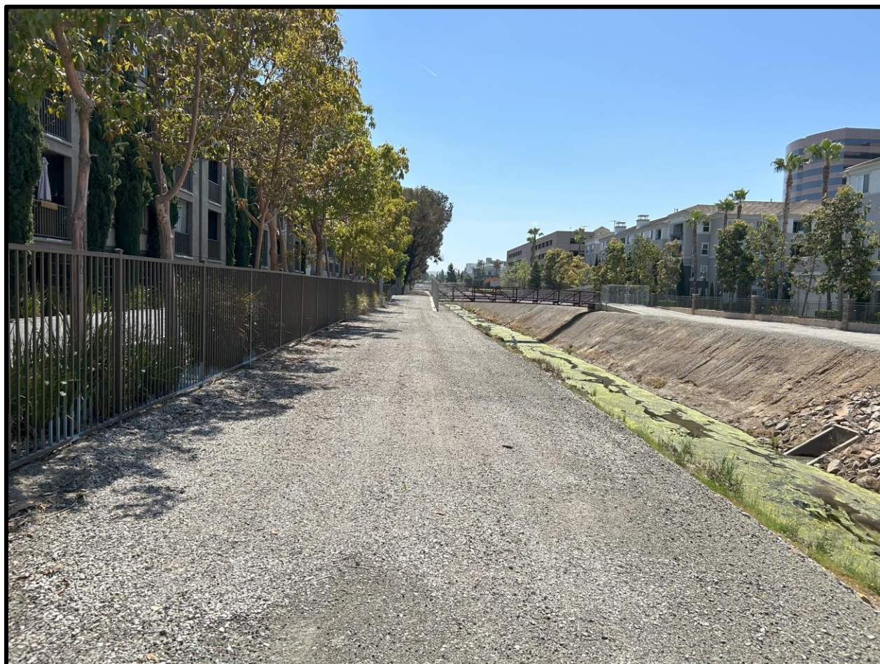
Figure 4.3-8 EAST (NORTH) BANK OF BARRANCA CHANNEL WITH PEDESTRIAN BRIDGE; VIEW TO THE SOUTHEAST TOWARD JAMBOREE ROAD
