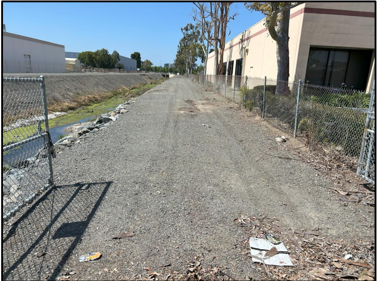
Figure 4.3-7 WEST BANK OF BARRANCA CHANNEL AND MAINTENANCE ROAD FROM SOUTH OF MCGAW AVENUE; VIEW TO THE SOUTH
