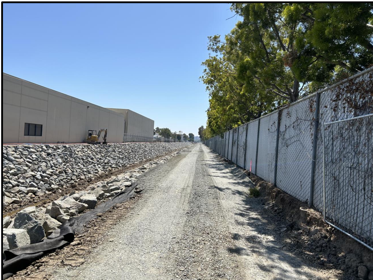
Figure 4.3-2 WEST BANK OF BARRANCA CHANNEL AND MAINTENANCE ROAD IN THE BARRANCA PARKWAY TO ALTON PARKWAY SEGMENT; VIEW TO THE SOUTH
