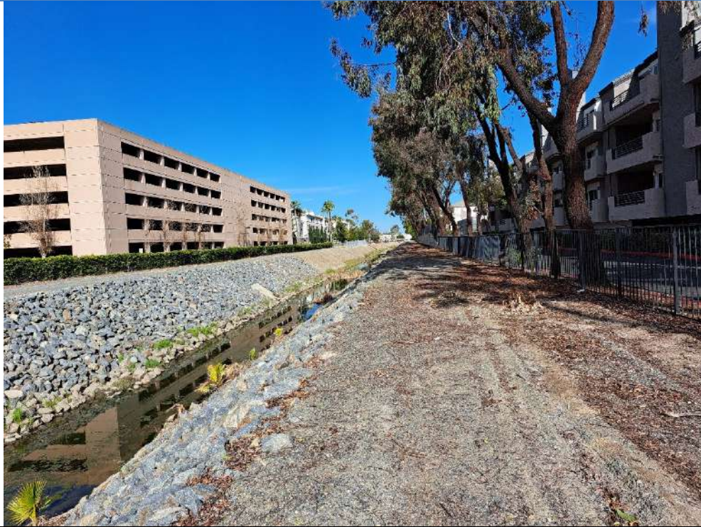
PHOTO 7: Partial view of Section C, looking west.
