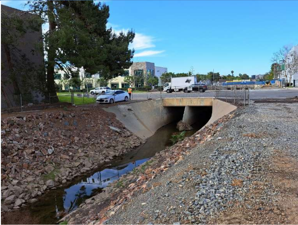
PHOTO 3: Partial view of Section A and Alton Parkway, looking south.
