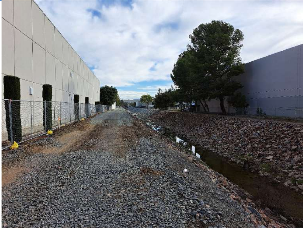
PHOTO 1: Partial view of Section A, looking north.
