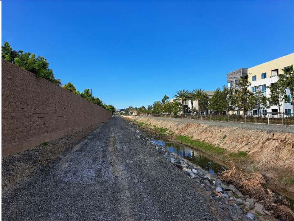
PHOTO 5: Partial view of Section B, looking south.
