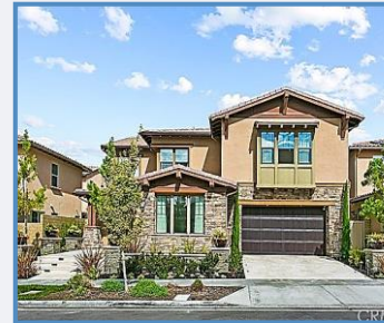
Medium Density (0 - 10 units/acre). Attached and conventional detached housing and other types of residential uses that have open space characteristics similar to single-family neighborhoods.
