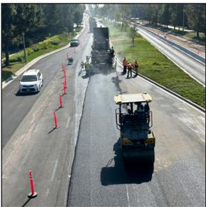
The project includes cold milling, roadway excavation, removal and replacement of asphalt pavement, concrete curb, gutter, curb ramps and sidewalks, utility protection, pavement delineation and signage, traffic signal modification, adjustment of
