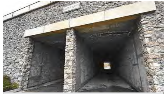
Jeffrey Open Trail Bridge
