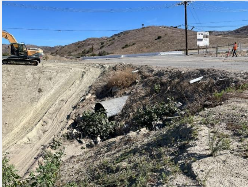
Photograph 8. Projecting corrugated metal outlet pipe of Map ID 4, view to the northeast
