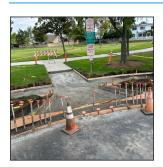
The One Irvine Improvements at Ranch Park includes the removal and replacement of concrete improvements and the construction of a new concrete pad with a shade structure to create a new picnic shelter area. The project is anticipated to be complete
