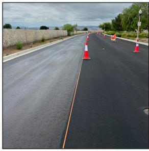
The street rehabilitation and slurry seal project along Pusan Way in the Great Park Neighborhood involves slurry seal rehabilitation, repair, and restriping between Irvine Boulevard and Cadence. The intent of the work is to improve roadway surface
