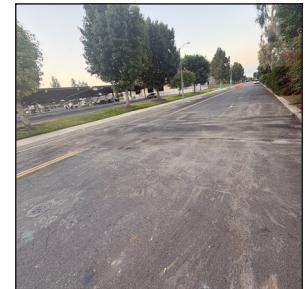
Escalar Avenue northwest of Irvine High School, were performed when school was not in session. The storm drain improvements involved trenching, installing pipe, and paving. The storm drain work has been completed and the remaining scope of this project
