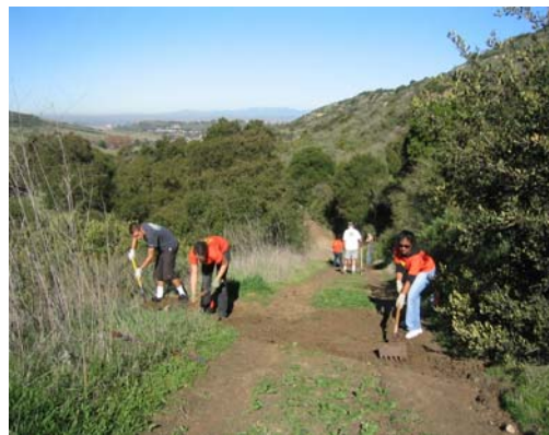
"Second Saturday" volunteers creating a water bar on the Bommer Canyon East Fork trail.
