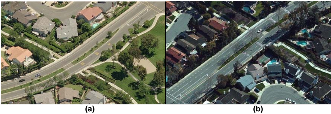
Figure H: Photos facing south of Venta Spur Trail at a) Westwood and b) Yale Ave
